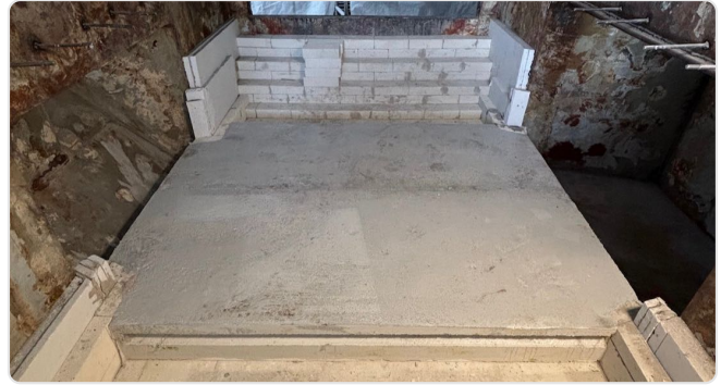
Bodembekleding met bekisting
