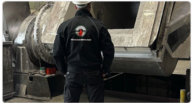
Charging chamber after refurbishment
