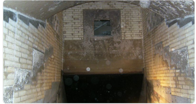
Ash and slag attack chemically and mechanically
