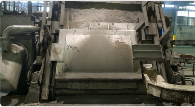
Anchor field before the castable is applied
