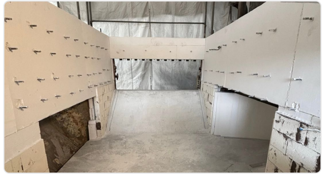
Anchoring in the hearth lining
