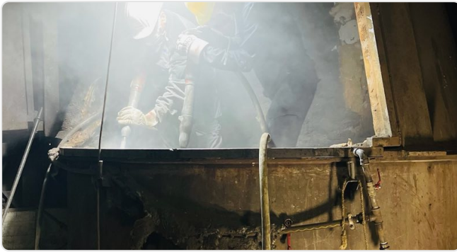
Cleaning and demolition before relining
