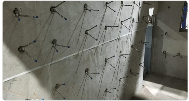
Rebuild: anchors in a grid on a new insulation layer
