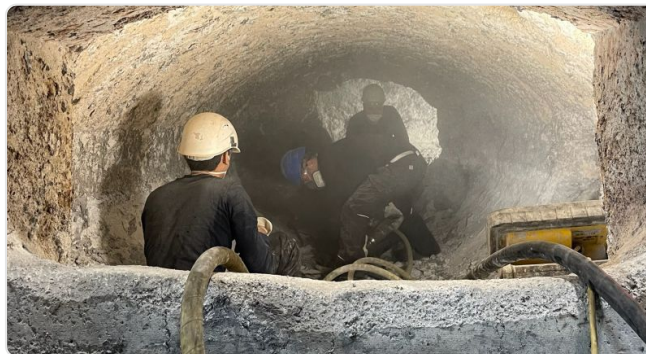
Maintenance gunning during the turnaround
