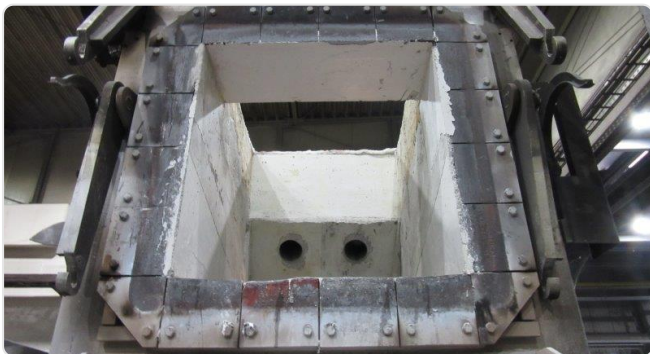
Burner lances after refurbishment
