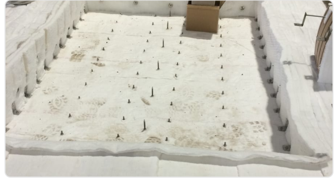
Anchor grid in the lid frame before casting
