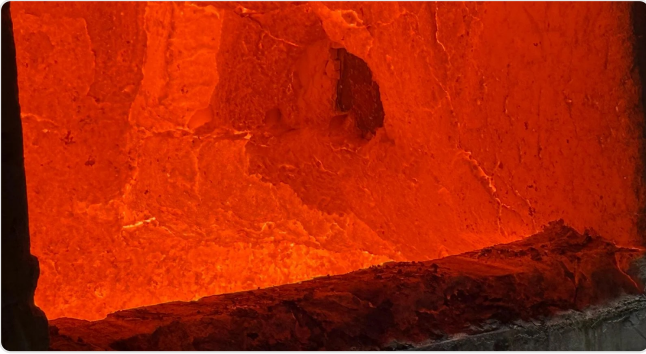
Emergency repair on an aluminium furnace
