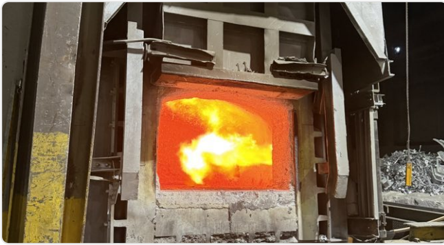
Relining in shift operation
