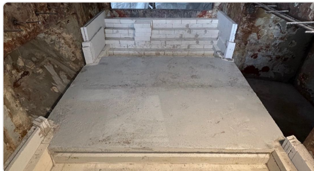
Hearth lining with formwork
