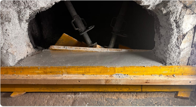
Charging opening: new hearth over formwork, angular spalling on the surround
