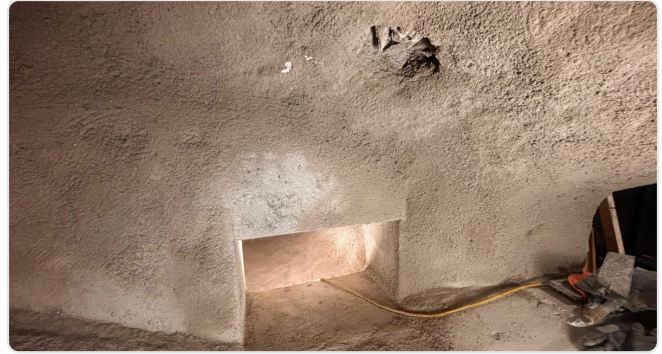
Monolithic wall and hearth in the area of the tool path
