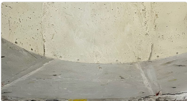
Finished monolithic lining with clean connections
