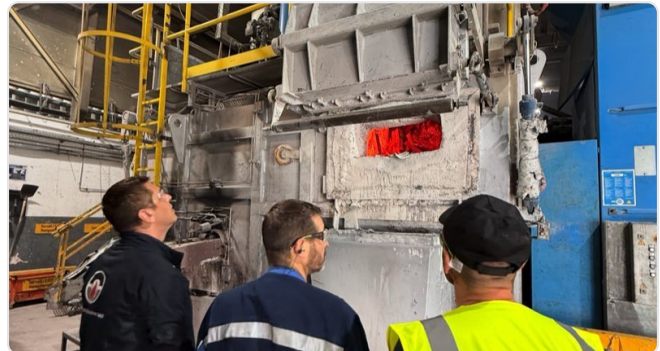
Inspection during shutdown
