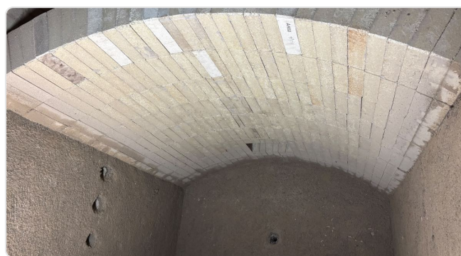
New arch in the combustion chamber
