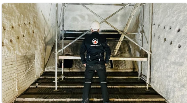
Lining of a wood-fired combustion plant
