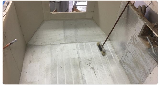
Lining with prefabricated shapes
