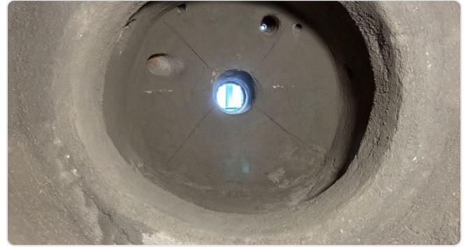
Expansion joint properly packed with fibre blanket
