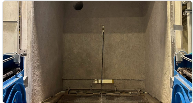
Fully lined hood before refitting
