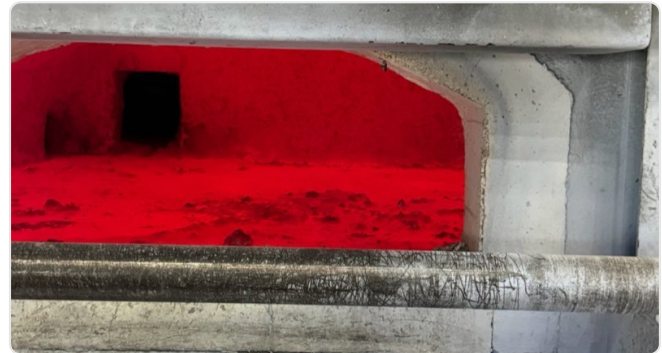
The bath line: the most heavily stressed band of the lining
