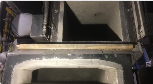
Complete overhaul of an aluminium melting furnace
