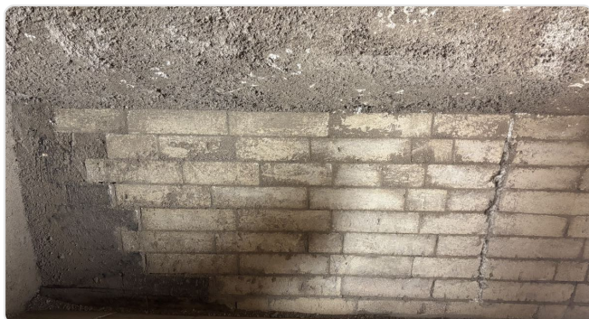
Stepped, interlocking transition, expansion joint on the right
